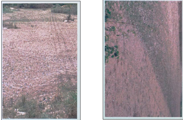
Figure 8: Leveling and releveling of ground
