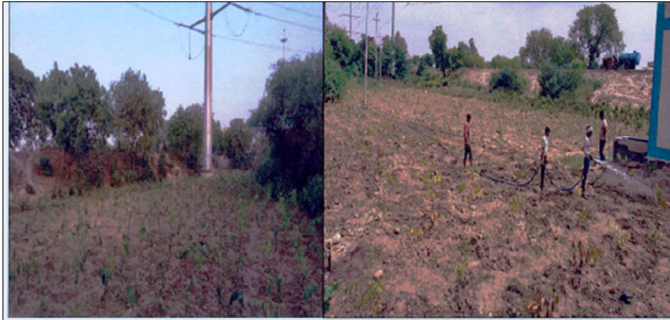
Figure 9: Leveling and releveling of ground
